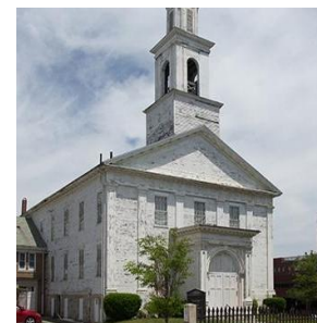
First Baptist Church, Restoration Project for Steeple Playhouse
